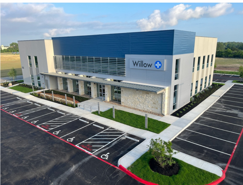
The Koehler Co. Guadalupe Regional Medical Center Willow Medical Office Building Healthcare Less than $10 Million
