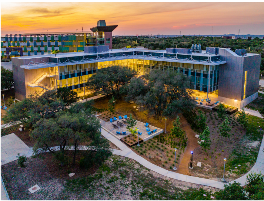
SpawGlass Contractors, Inc. Northwest Vista College STEM Building Institutional $10 to $25 Million
