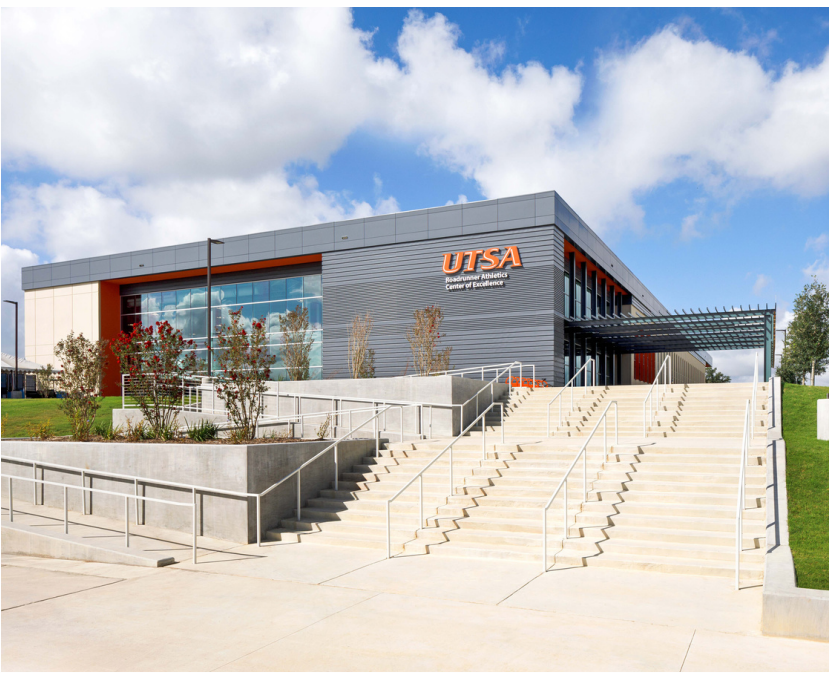
Joeris General Contractors, Ltd. UTSA Roadrunner Athletics Center of Excellence Institutional $25 to $100 Million
