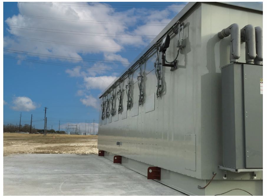
Alpha Building Corporation Decker Creek Power Station Control Center Buildout - Phase 1 and 2 Industrial: Less than $5 Million Community/Public Service
