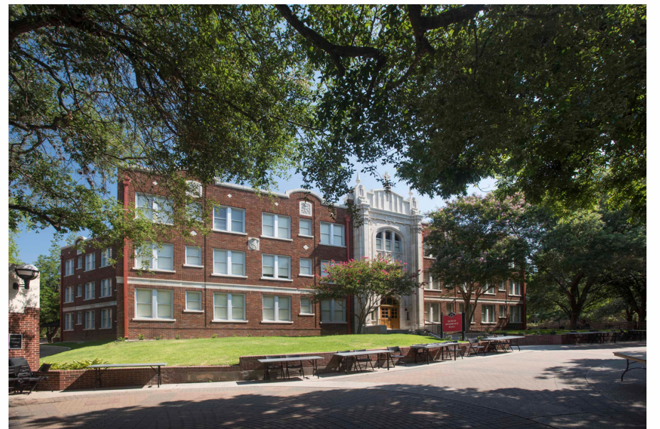
Joeris General Contractors, Ltd. University of the Incarnate Word Dubuis Hall Historical Restoration $2 to $10 Million
