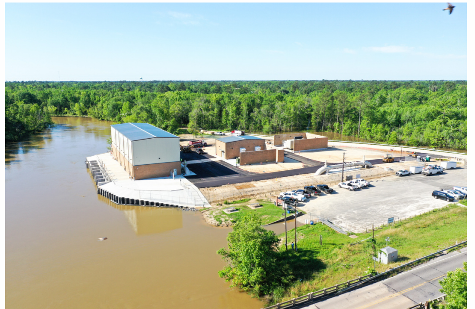
Garney Companies Sabine River Authority Pump Station and Pipeline Public Works/Environmental All Contract Amounts
